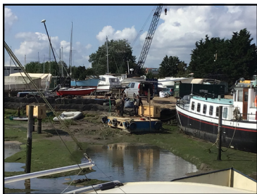
Robertsons pontoon work underway.
